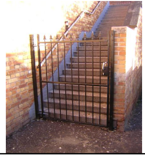
One of the two new gates installed at the sides of the shops in Chandag Road
